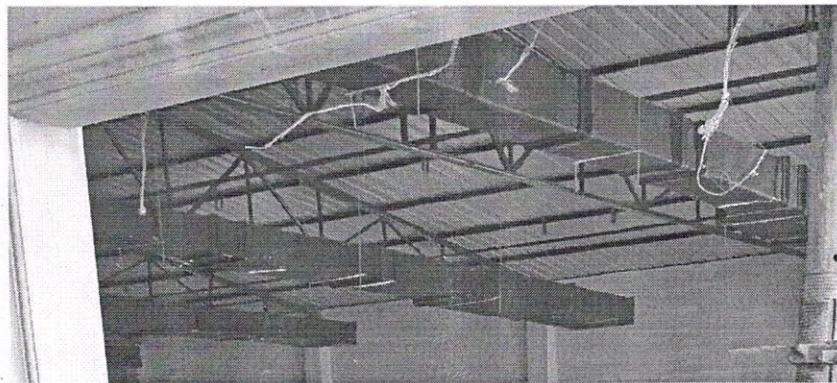
Truss elements arrangement for function hall
